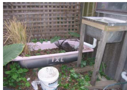
Right: Outside the laundry is an old trough taking the grey water from the washing machine. The grey water then runs into a bath with plants to filter the water. From there it goes into an underground pipe and is gravity fed to a bog garden in the front yard.
